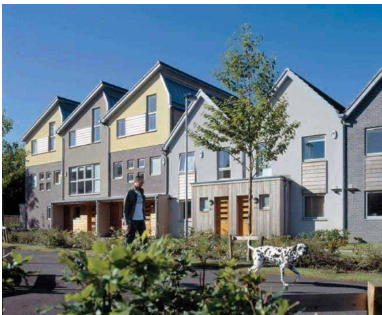
Even Wimpey can get it right – Staiths, Gateshead
