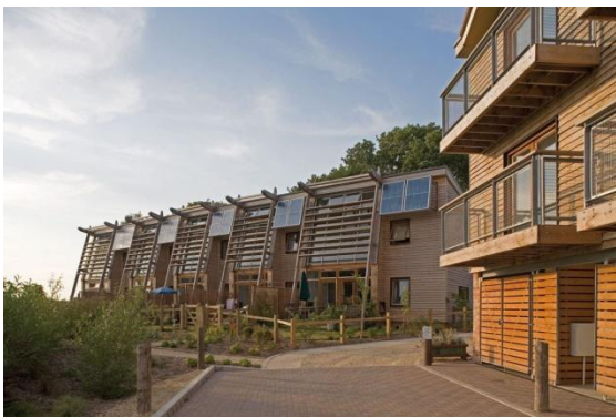
Low energy development –Langport, Suffolk
